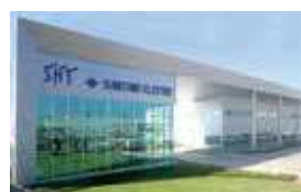
P9 Sumitomo Electric Hardmetal Manufacturing (Thailand), Ltd.
